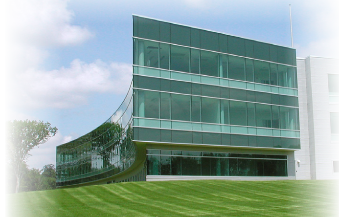
North American Headquarters, Mahwah, NJ
